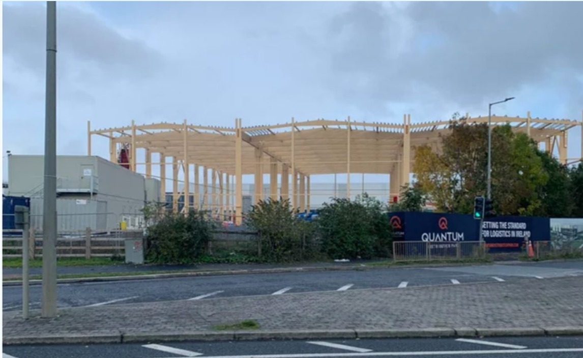
Figure 4.1: Warehouse under Construction in Blanchardstown Using Timber MMC
